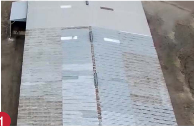
Rusty metal roof prior to restoration work.
