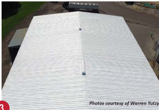
Metal roof after Benchmark® acrylic top coat.
