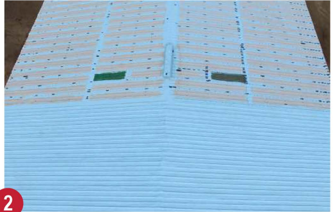
Metal roof after application of Spunflex® fabric and Benchmark® base coat to the seams along with Kwik Kaulk® sealant application to the fasteners.
